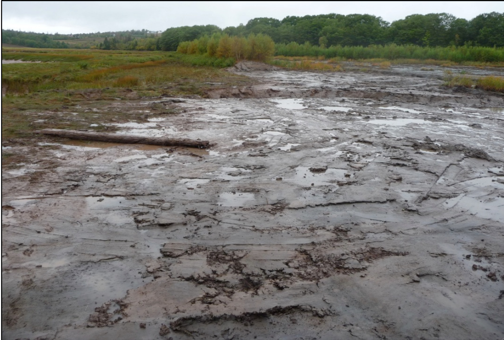
Figure 5 Completed breach (60 m) and tide channel. Photograph by T. Bowron, 24 September 2009.
