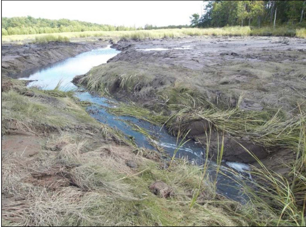
Figure 6 Tidal channel following completion of restoration work (looking from mouth of channel towards interior of the restoration site). Photograph by J. Graham, 23 September 2009.
