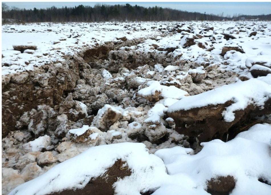
Figure 4 Channel and dyke breach. Photograph from the fringe marsh near the mouth of the channel looking towards restoration site.
